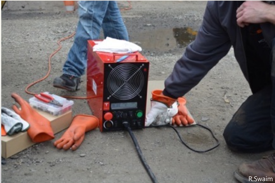
Factory provided resistor bank could not reach isolated modules
