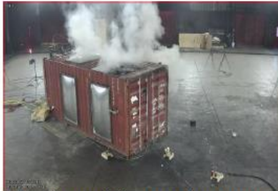
Continued thermal runaway propagation [TR + 00:46:26]
