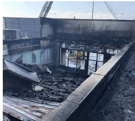
(b) From Adjacent Roof
