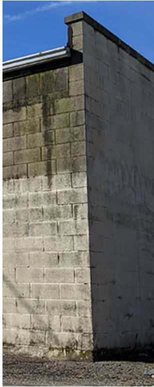
(a) Masonry Block Wall
