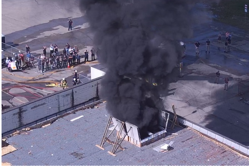
Figure 3.64: A drone image of the roof vents looking from the CD corner toward the AB corner 30 s after the initial suppression (9 min 54 s after ignition) in Experiment 6.
