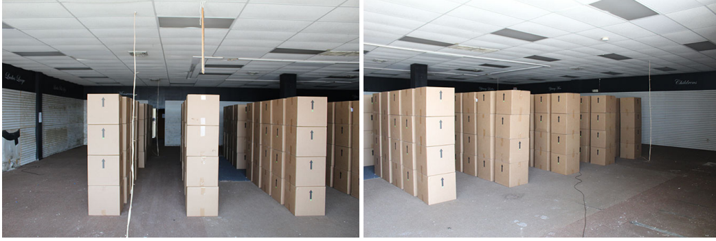
Figure 2.14: Images of the interior of unit 1069–1071. Looking toward the AB corner from the front entry door (left), and looking toward the CD corner from the front entry door (right).
