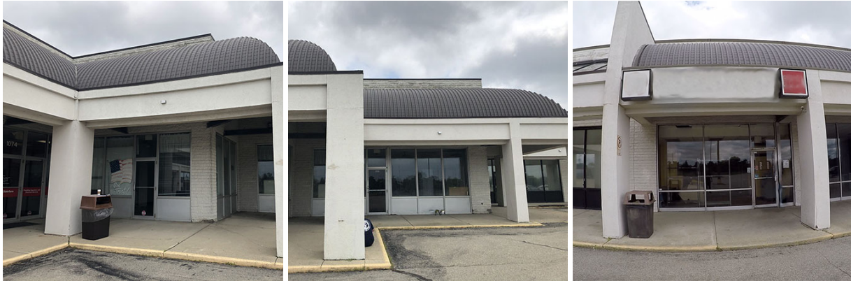
(a) Unit 1076 Entrance 1
