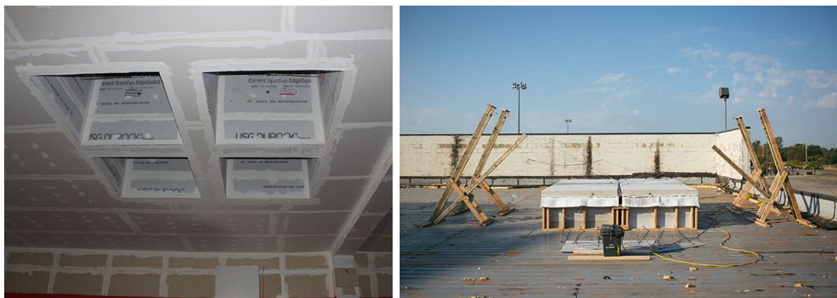
(a) Underside of Roof Vents
