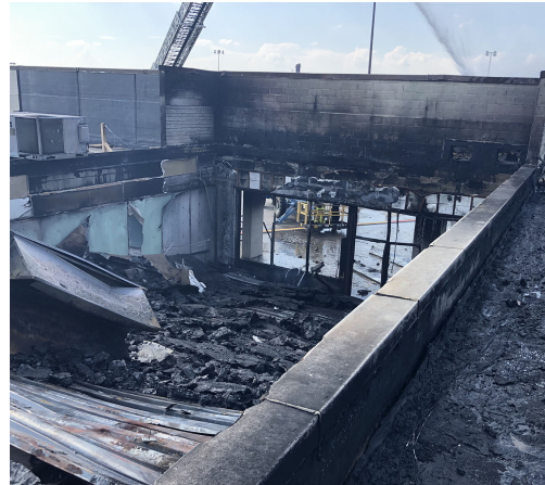
(b) From Adjacent Roof
