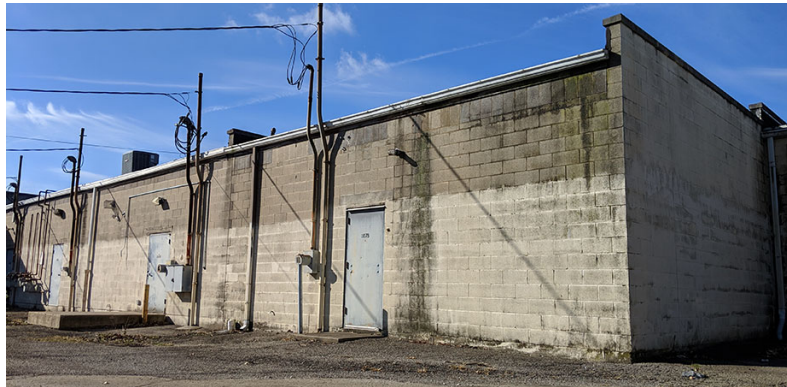
(d) Side C (Example of Typical Rear of Units)
