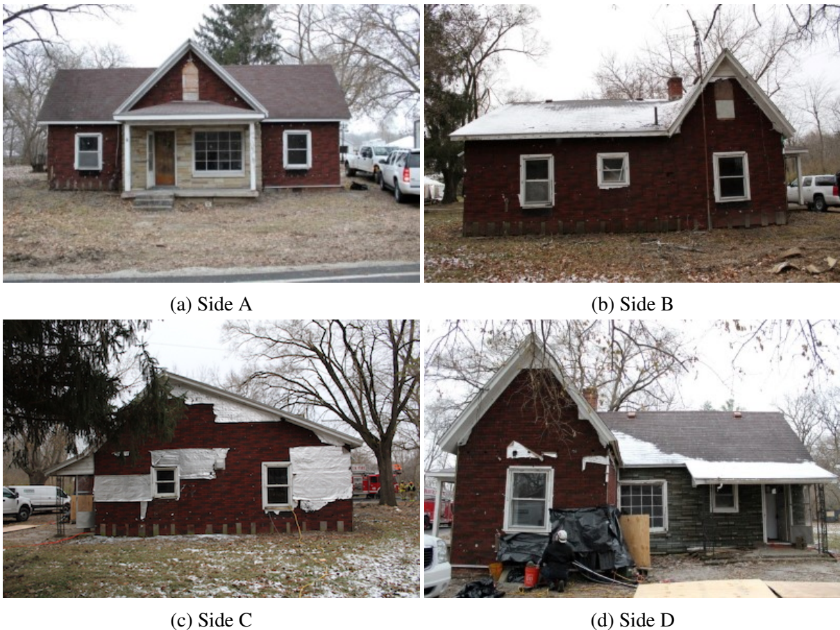
Figure 3.187: Exterior photographs of the structure for Experiment 16.
