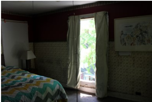
(c) C/D Corner Wall
