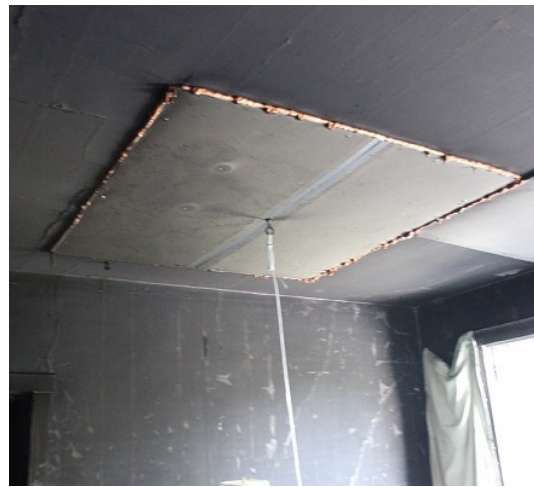
(b) Interior Ceiling
