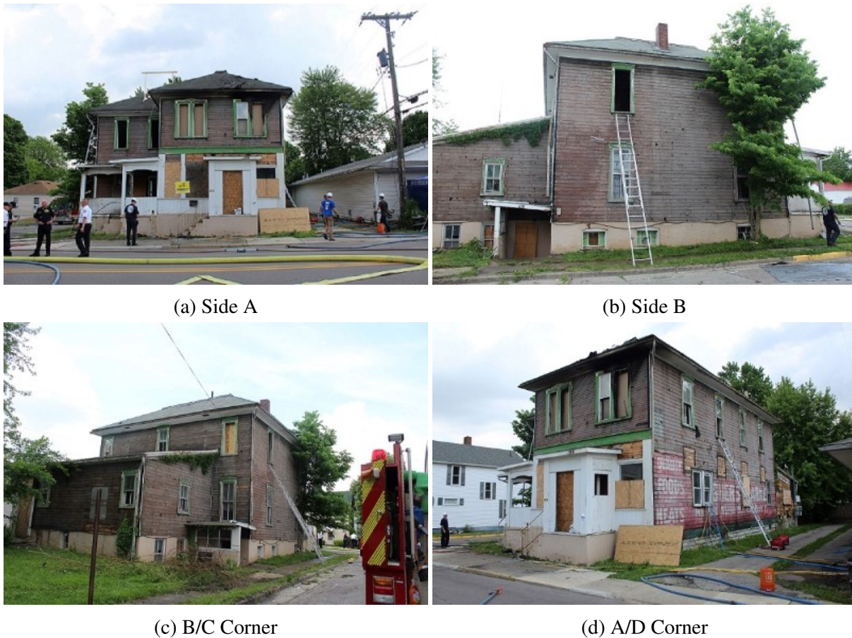
Figure 3.86: Exterior photographs of the structure for Experiment 8.
