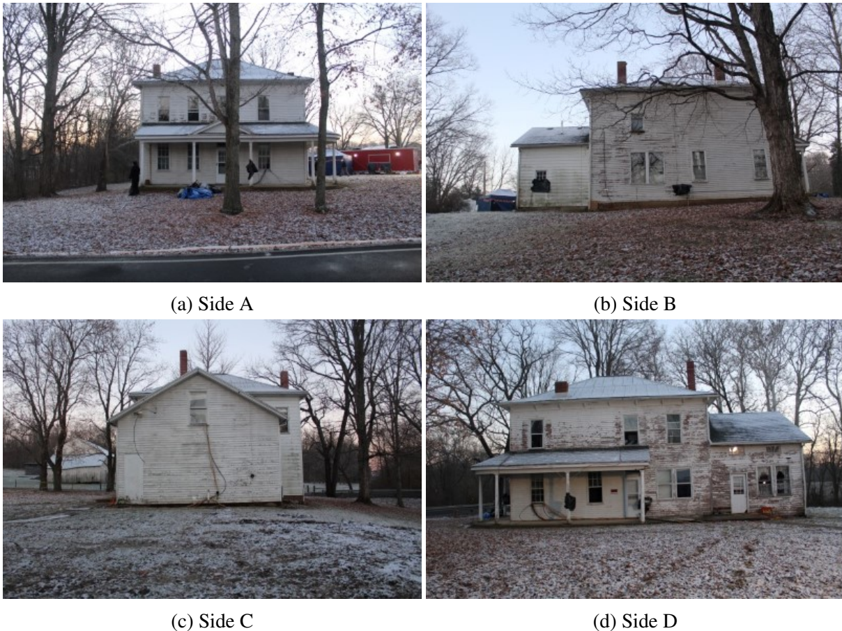
Figure 3.61: Exterior photographs of the structure for Experiment 6.
