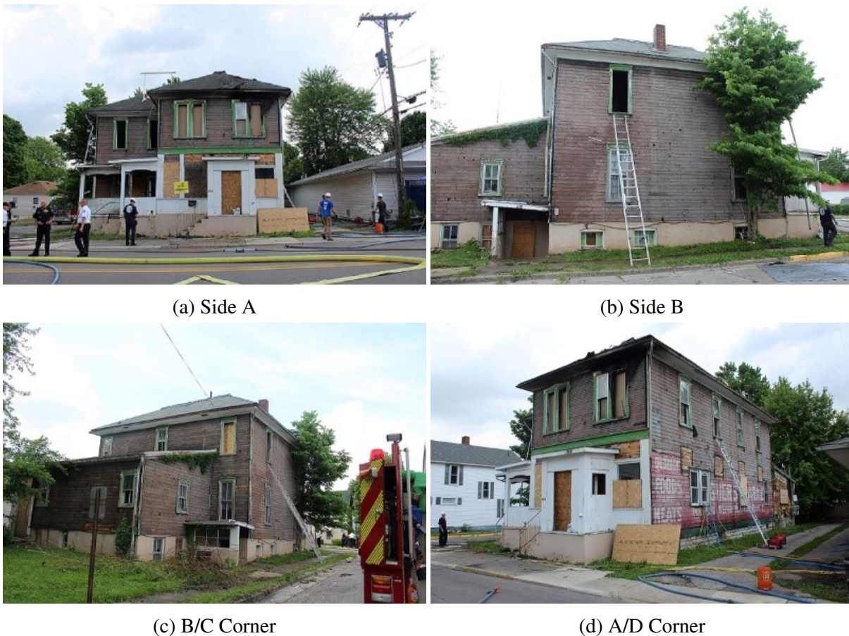
Figure 3.72: Exterior photographs of the structure for Experiment 7.
