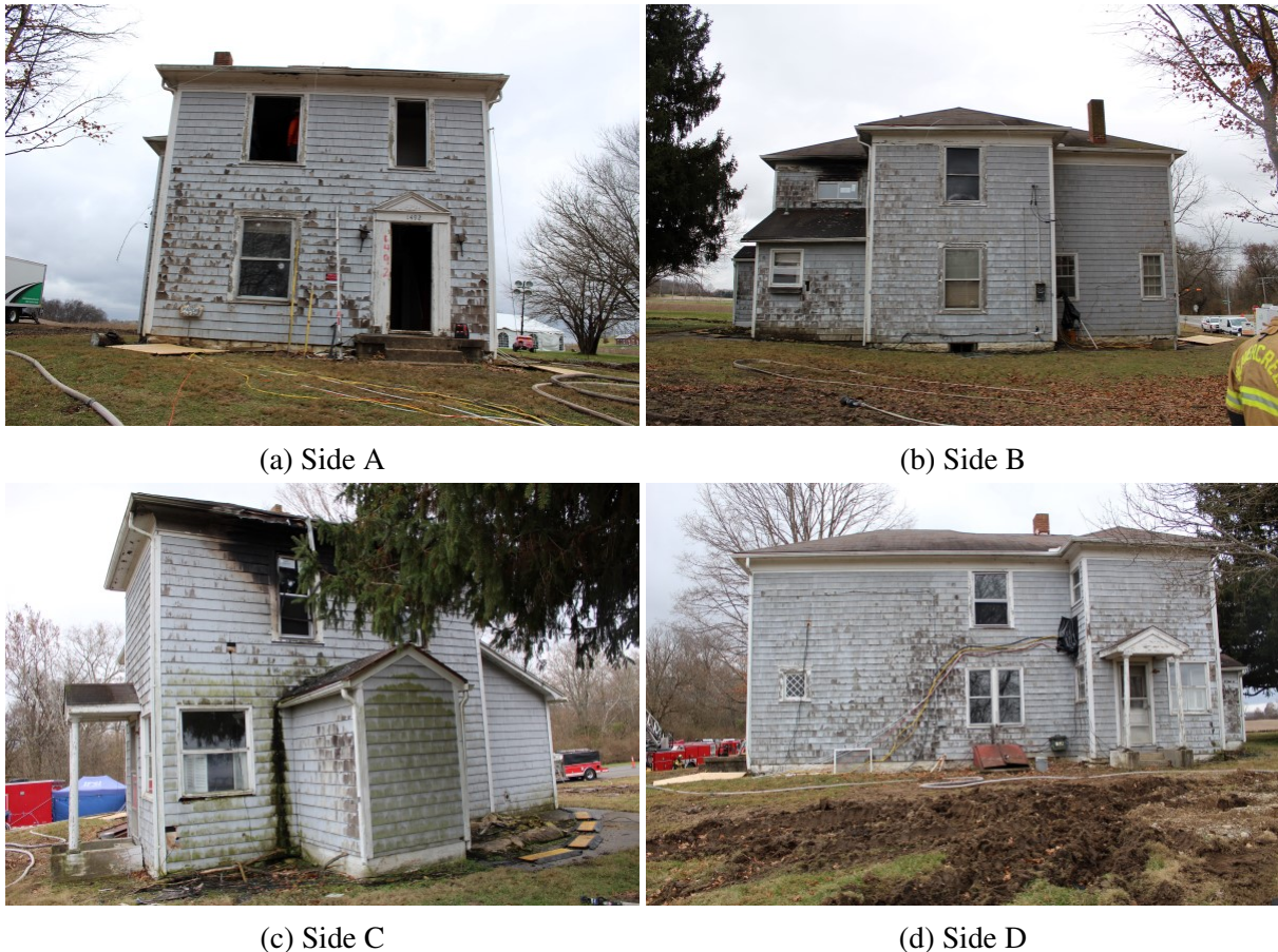
Figure 3.148: Exterior photographs of the structure for Experiment 13.
