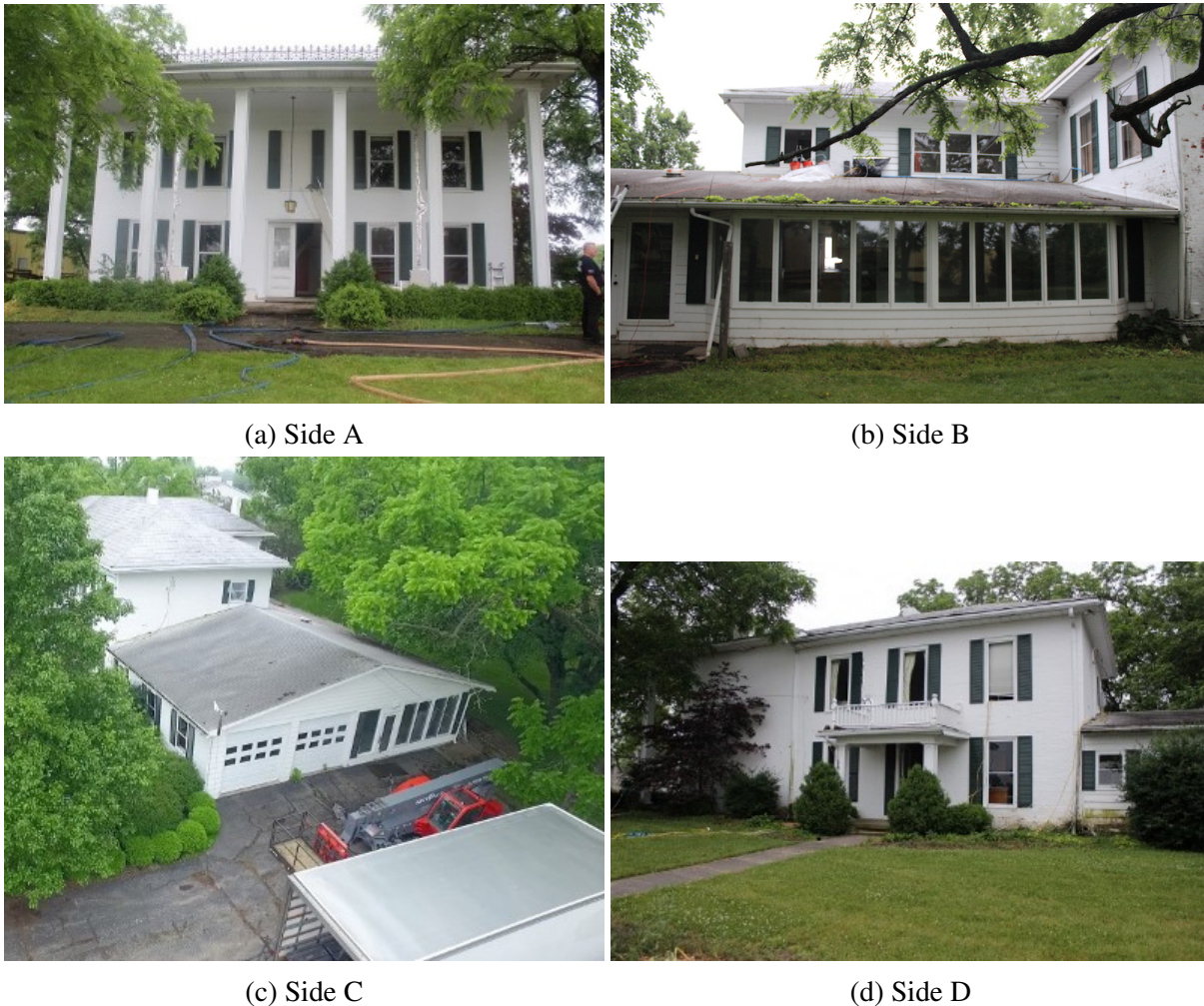
Figure 3.39: Exterior photographs of the structure for Experiment 4.
