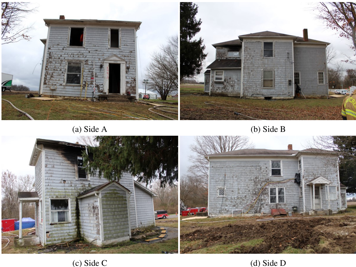
Figure 3.26: Exterior photographs of the structure for Experiment 3.
