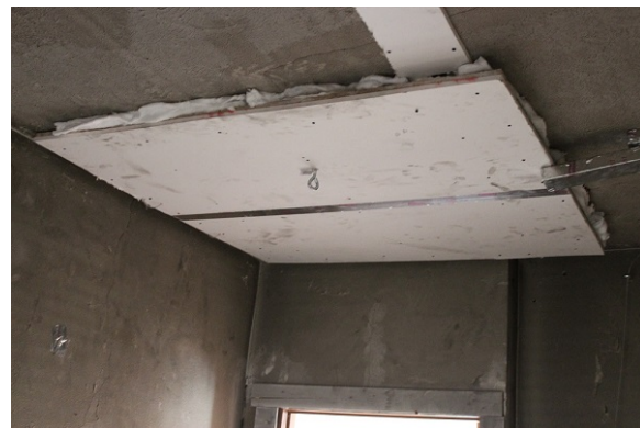
(b) Interior Ceiling
