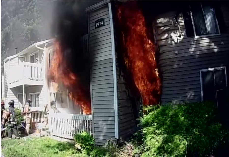
Figure 3.96: An image of fire growth prior to opening exterior door (999 s).
