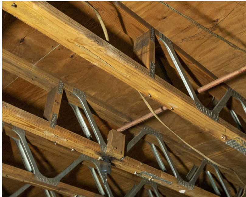
Figure 2.4: A view of the underside of the floor construction.
