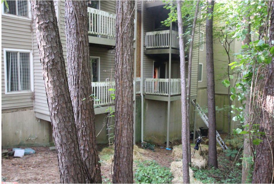
Figure 5.31: Rear elevation of the fire building for Experiment 5, pictured shortly after ignition.
