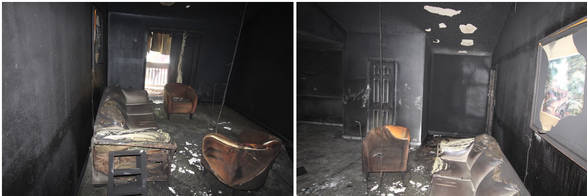
Figure 4.26: Pyrolyzed furniture located in the living room of Apartment F during Experiment 5.
