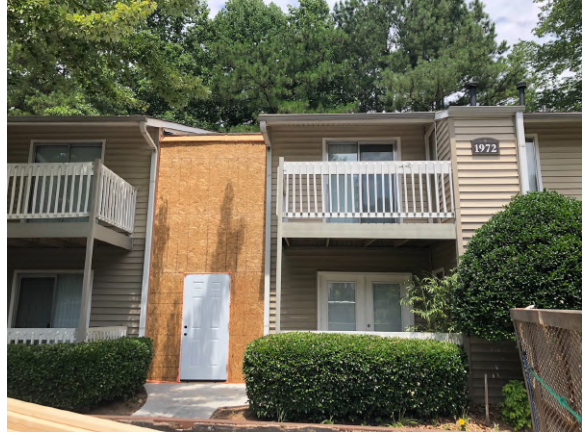
(b) Exterior of Breezeway
