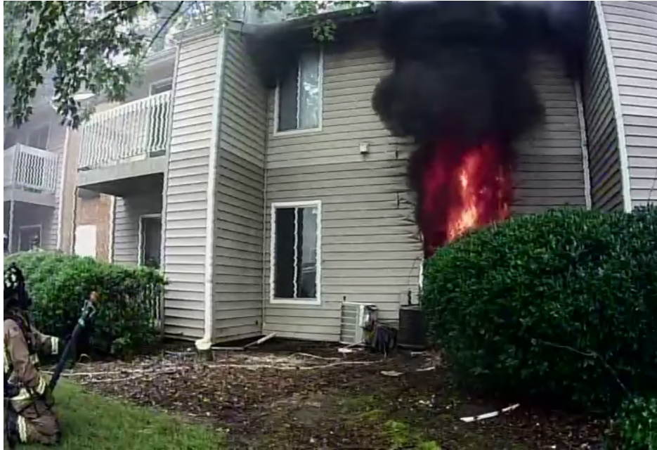
Figure 3.79: Image of the fire room (bedroom) window when the exterior breezeway door was opened in Experiment 2B.
