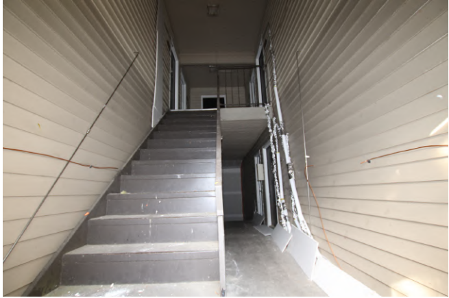
(a) Interior of Breezeway, Stairs to Second-Floor
